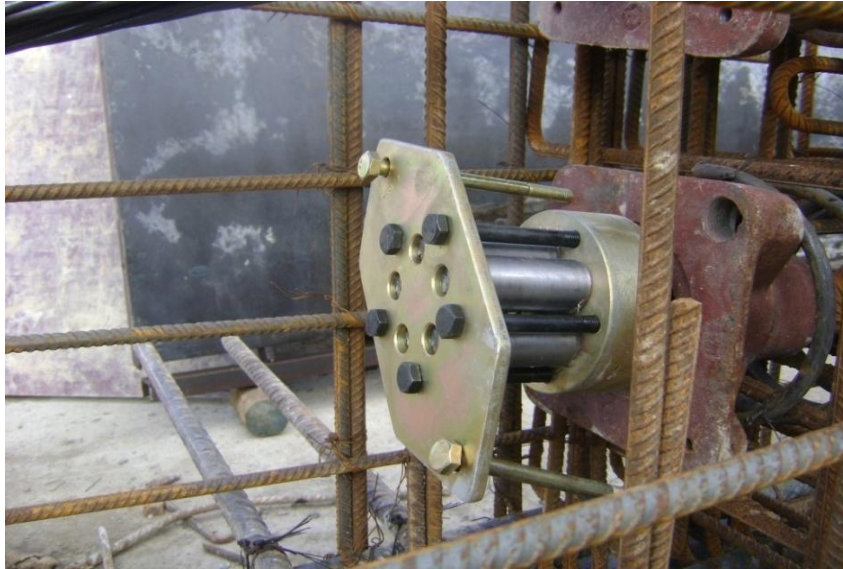
Figure I-7 : Plaque d'ancrage (ancrage passif).
