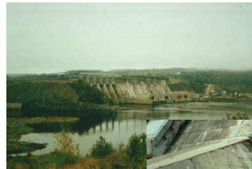
Slot Cutting at Mactaquac G.S. New Brunswick
