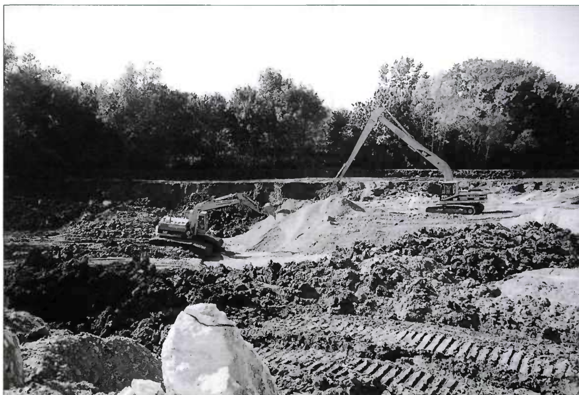
Autoroute A 89 – Section 1 – LRPC Bordeaux
