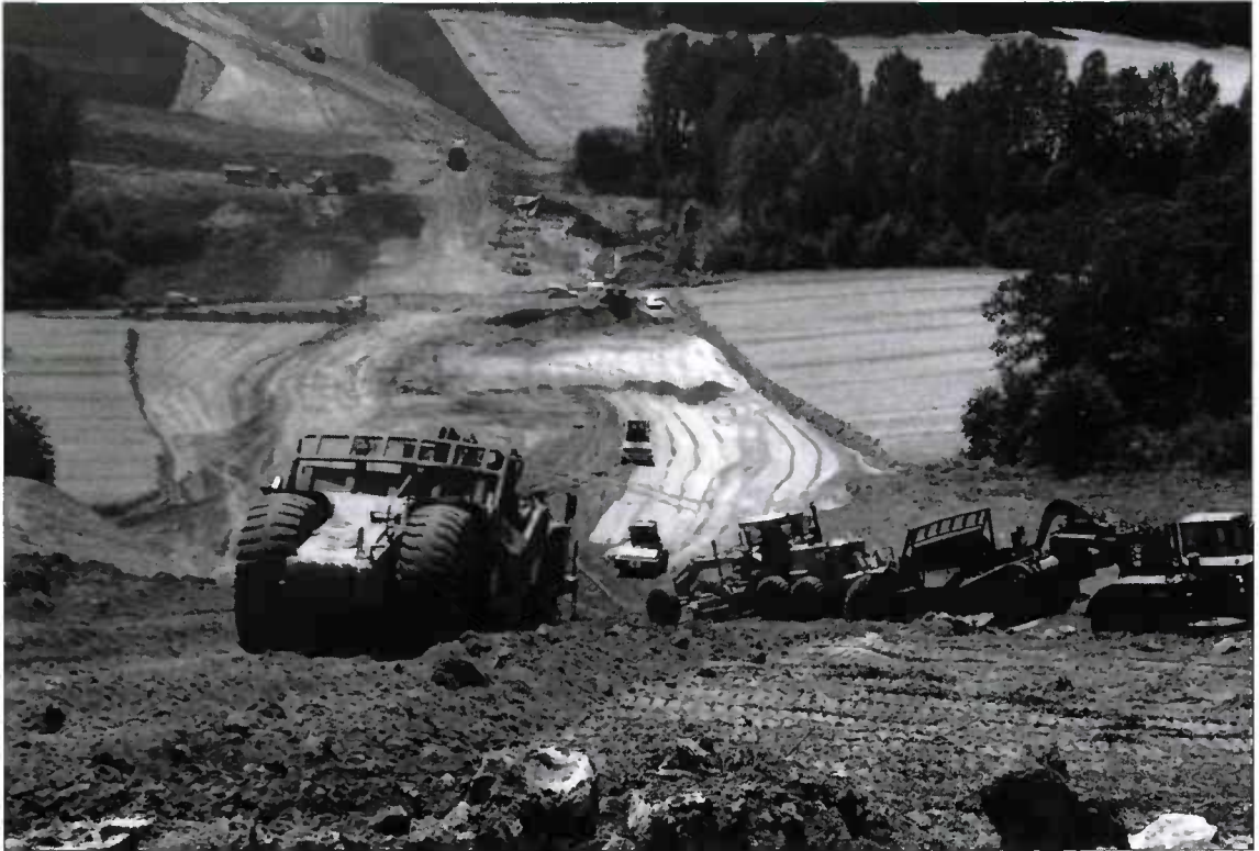
RN 32 - Compiègne-Ribecourt - Photo LRPC Saint-Quentin
