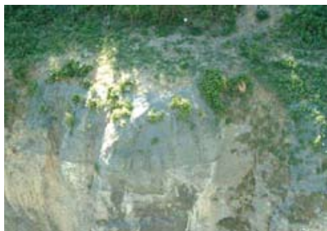
▲ Figure 58 : filets PVC plaqués [RiskYdrogeo]
