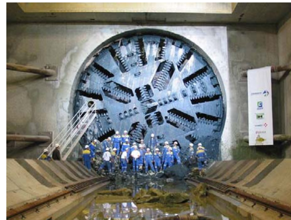
SOCATOP – Percement VL1
