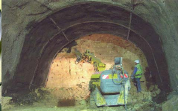
Niche Tunnel SOCATOP
