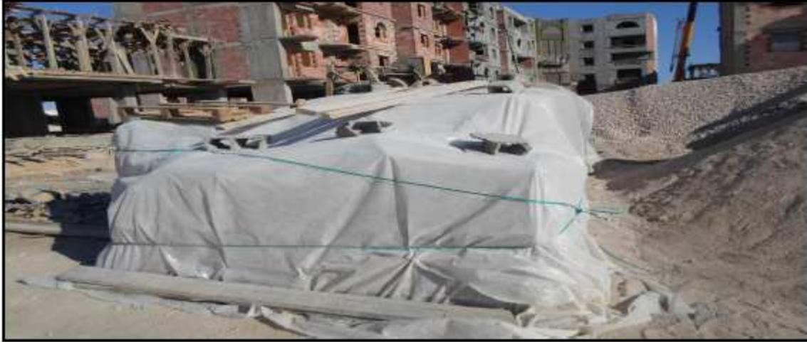
Figure 21 : stockage du ciment
