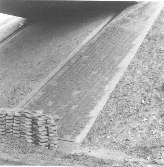
figure 35 Mise en oeuvre des dallettes (pavés Trief).
