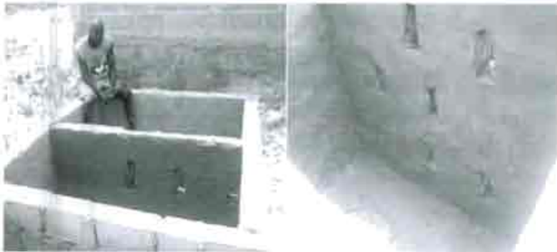
Figure 5: Fosse septique en construction
